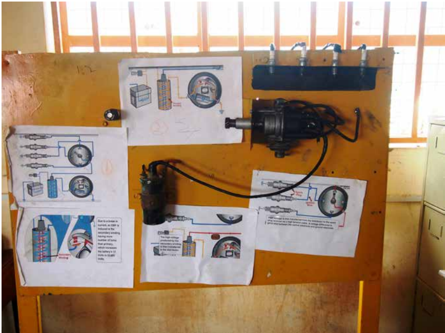
Figure 3.2. Norwegian Refugee Council electrical-training centre: practice board in electrical class in Kakuma, Kenya. © Sarah Rosenberg-Jansen.
