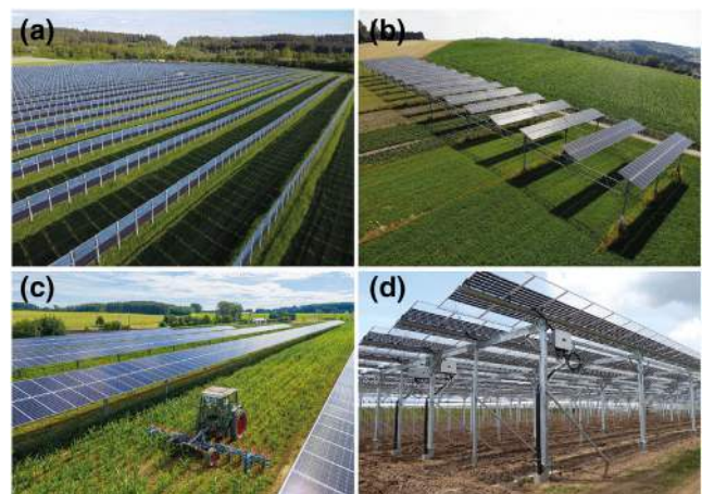
FIGURE 1 Different types of agrivoltaic systems. (a) Vertical system on grassland—farming between solar panels (Donaueschingen-Aasen, Germany, image credit: Next2Sun), (b) system with clear height on arable land—farming under solar panels (Herdwangen-Schönach, Germany, image credit: BayWa r.e.), (c) ground level system on arable land—farming between solar panels (Althegenberg, Germany, image credit: Matthias Baumgärtner Videofotografie/ÖKO-HAUS), (d) system with clear height in orcharding—farming under solar panels (Ahrweiler, Germany, image credit: Fraunhofer ISE).
