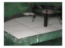
Typical gas stoves connected to biogas latrines in Nairobi (top) and Kampala (bottom).
