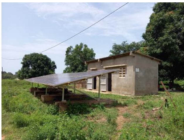
Figures 1 and 2. An ERSEN mini-grid, with its 24 solar panels, battery and inverter storage room (left) and diesel generator (right)
